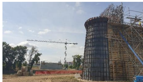
Figura 2. Cofraj metalic special
